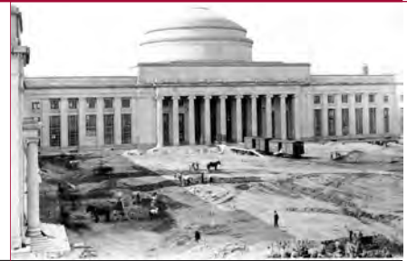
Constructing the Dome (see p. 8)
