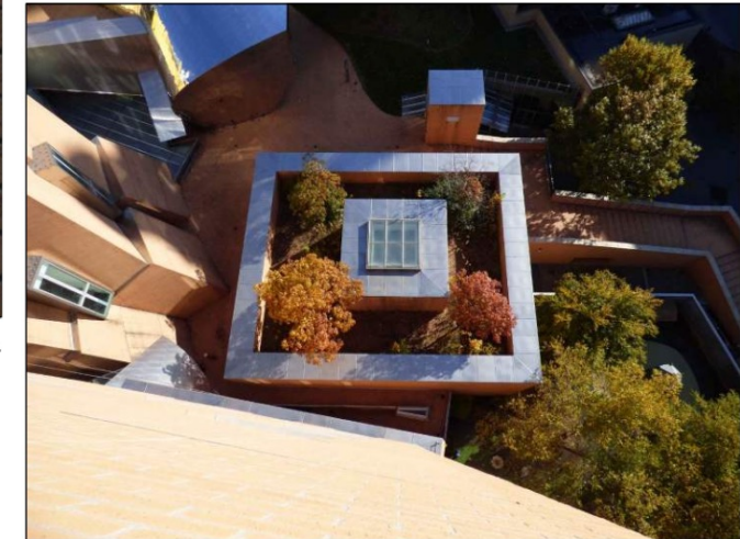
STAINLESS STEEL COPING AND ROOF AT LECTURE HALL 123
